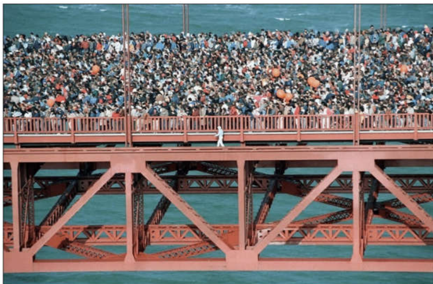
Golden Gate Bridge on its 50th Anniversary in May 1987: a classic example of live loads overload AP Photo / Doug Atkins
